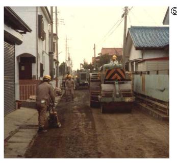
\*After grading work by a grader, etc, the new paving course is compacted sufficiently by a roller. In case the mixing thickness is more than about 20cm, additional employing of a large size vibrating roller is preferable.
