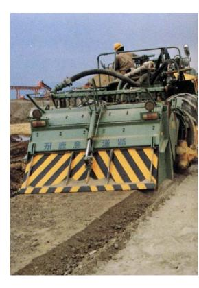
\* The work of crushing, agitating and mixing is concurrently carried out by Super Stabilizer.
