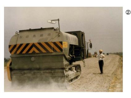
\* Spreading a prescribed amount of stabilization agent onto an existing pavement surface.
